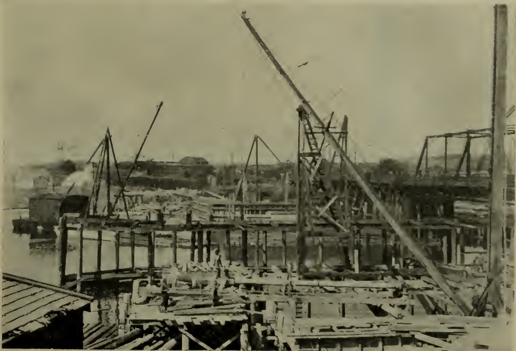
FIG. 10. GENERAL VIEW FROM EAST.
